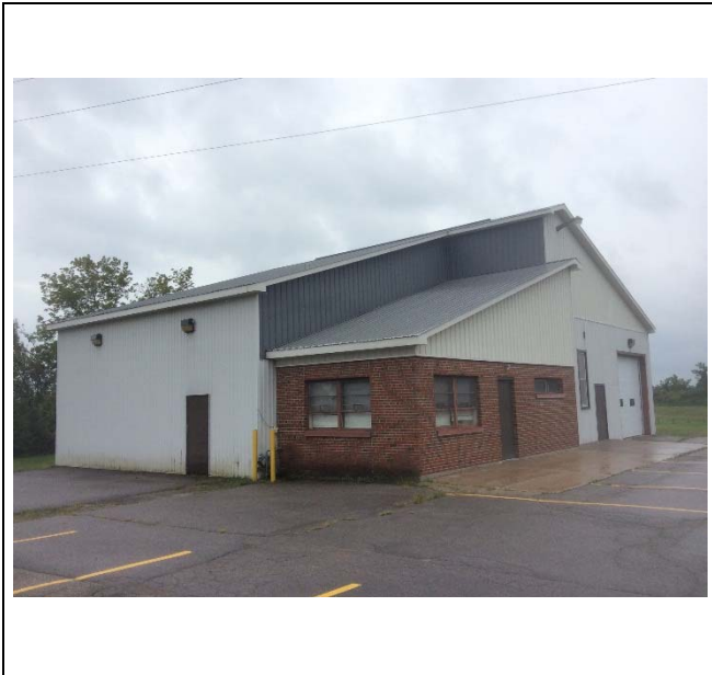
Photo 1: General view of the building.
