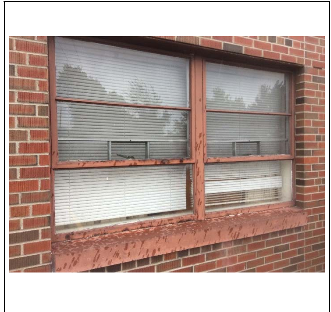
Photo 2: Window with steel frame.
