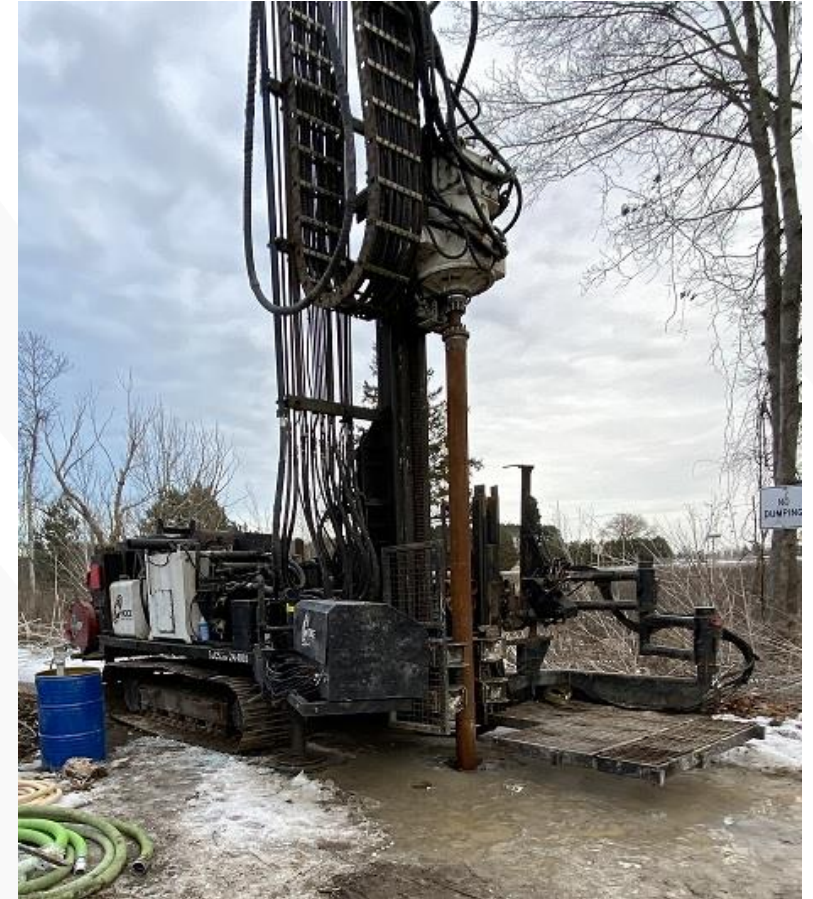
Monitoring well installation, McDowell Road
