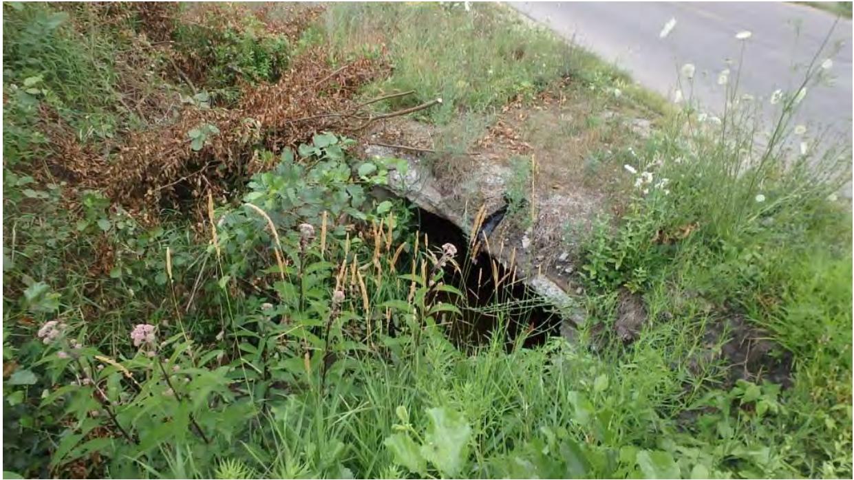
Figure 3 Outlet, Small Culvert
