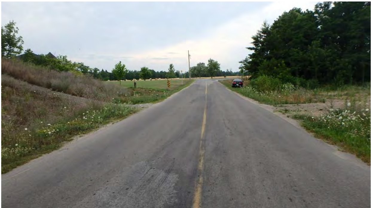
Figure 2 South Approach, Note Structure Removed
