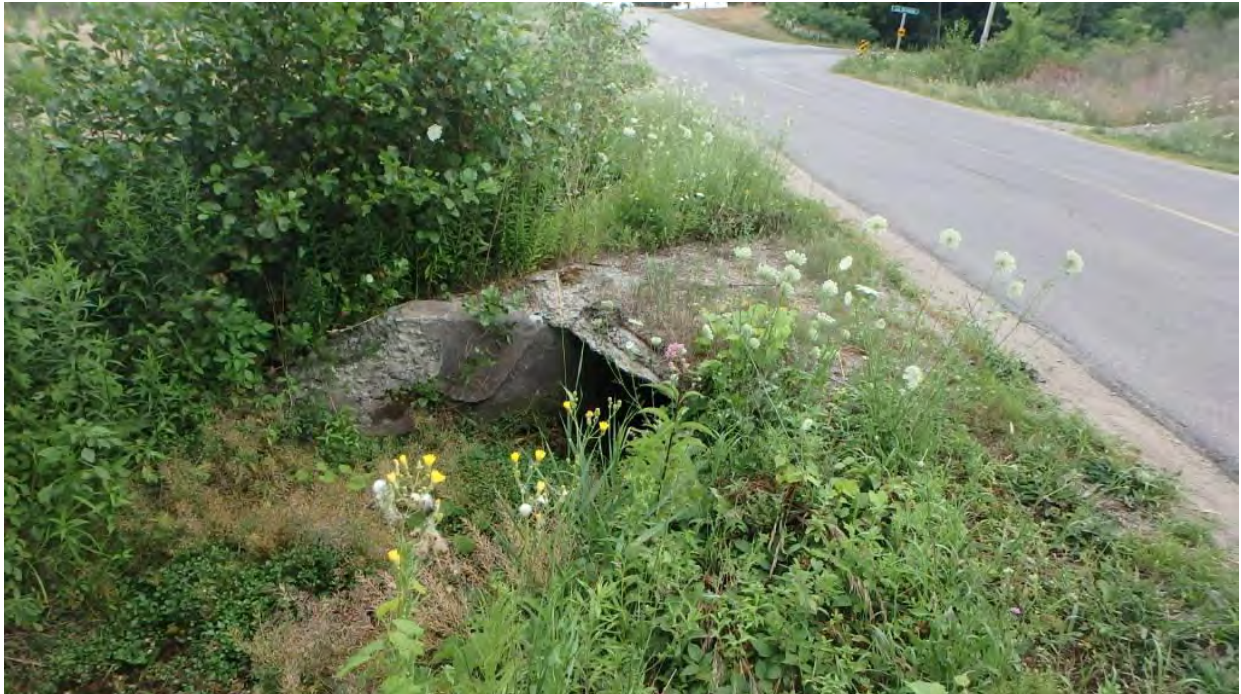
Figure 4 Inlet, Small Culvert
