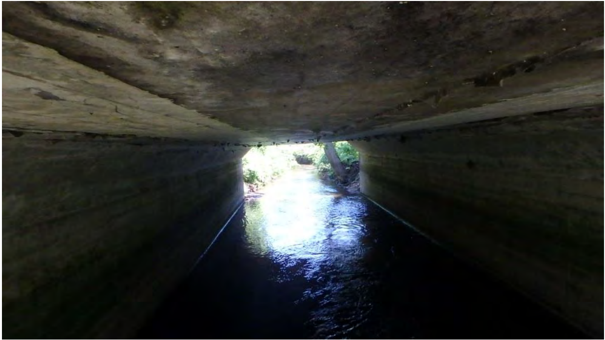
Figure 7 Barrel, Looking South
