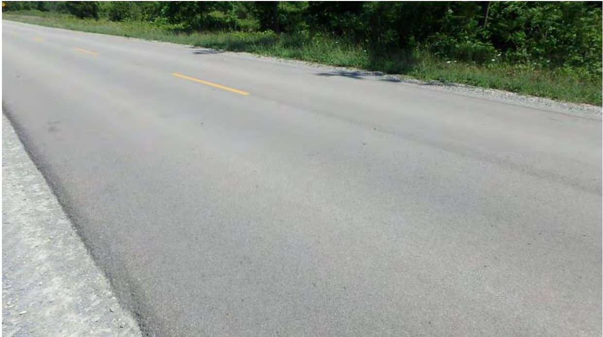
Figure 12 New Asphalt Wearing Surface
