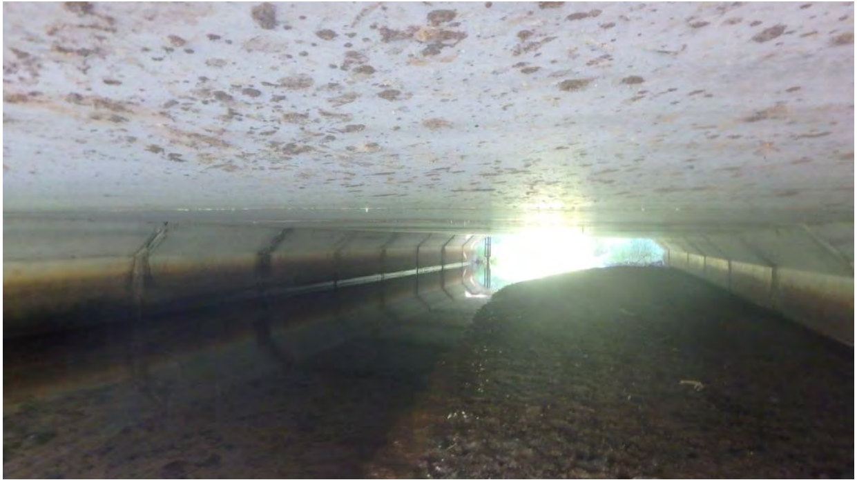
Figure 7 Barrel from East
