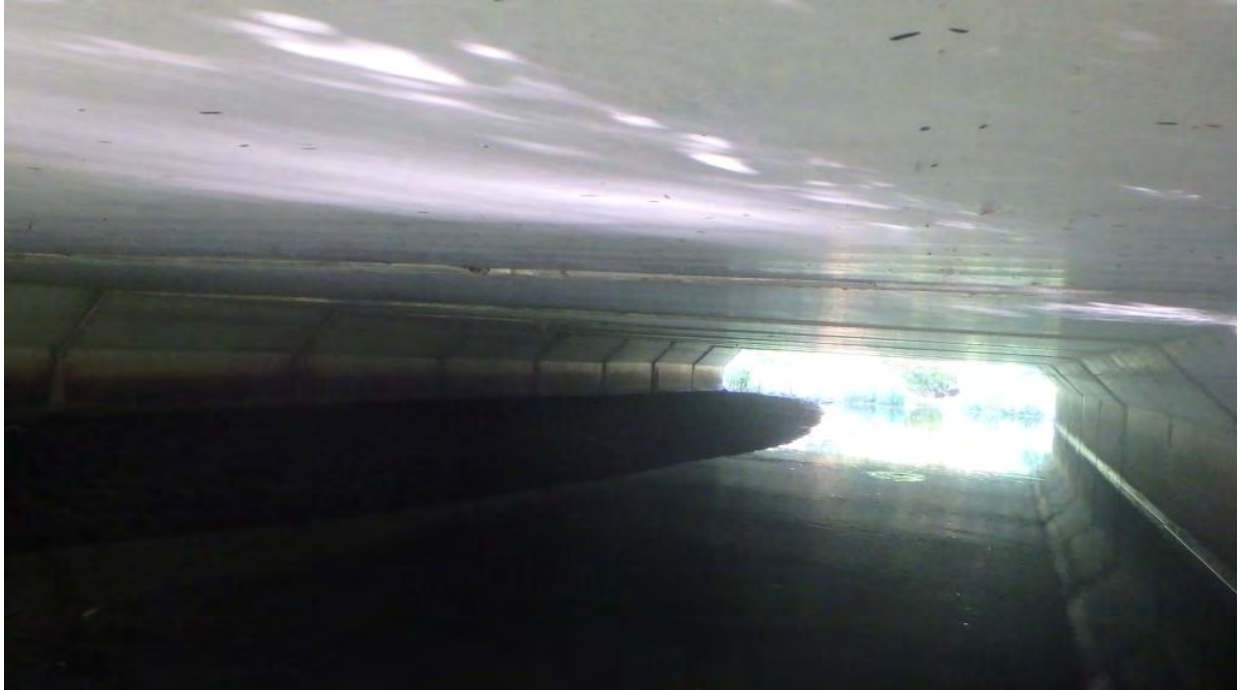
Figure 8 Barrel from West
