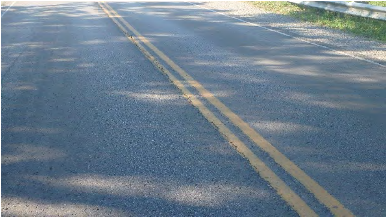
Figure 13 Longitudinal Crack in Wearing Surface Centreline
