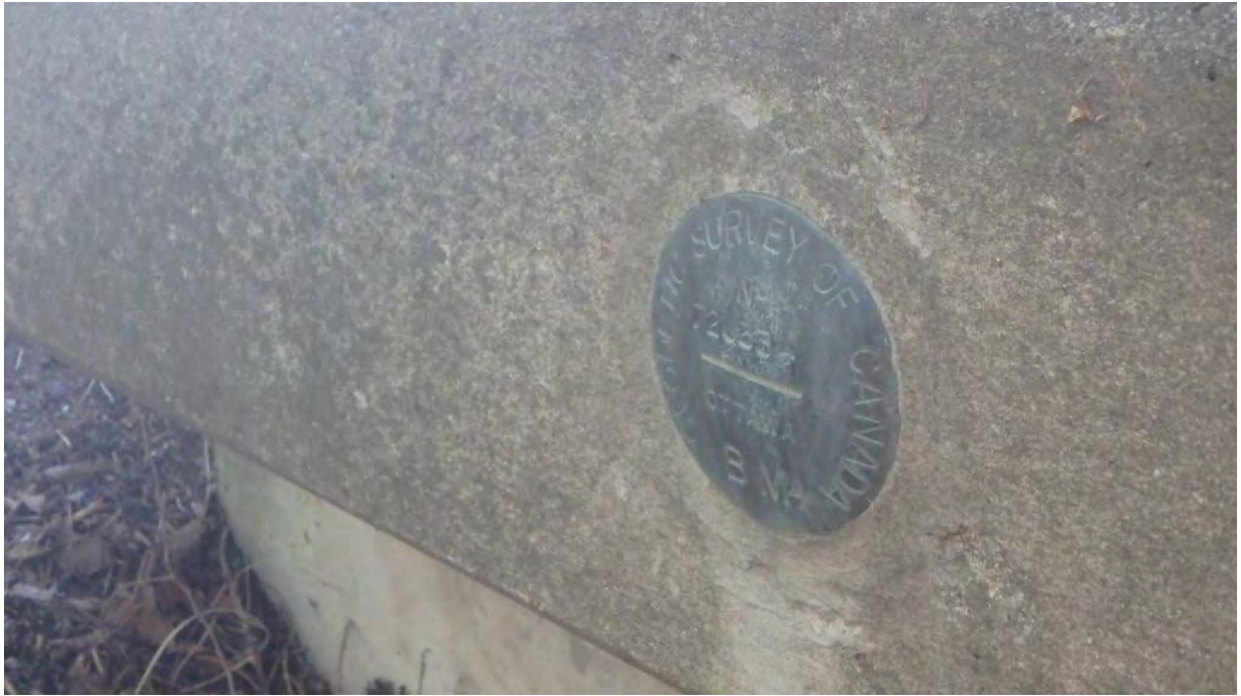
Figure 14 Geodetic Benchmark on West Fascia
