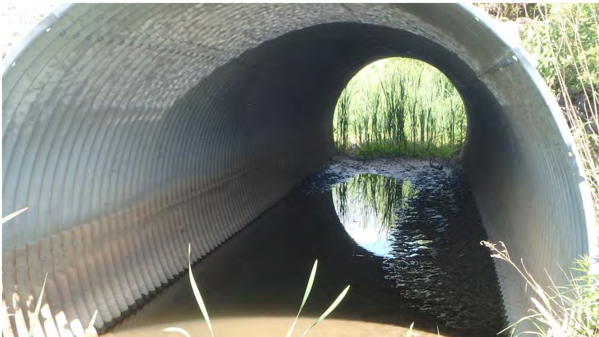
Figure 8 South Barrel, Looking East
