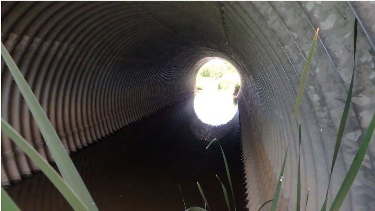
Figure 7 North Barrel, Looking West
