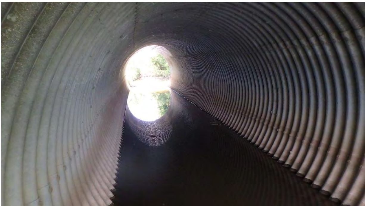
Figure 8 South Barrel, Looking West
