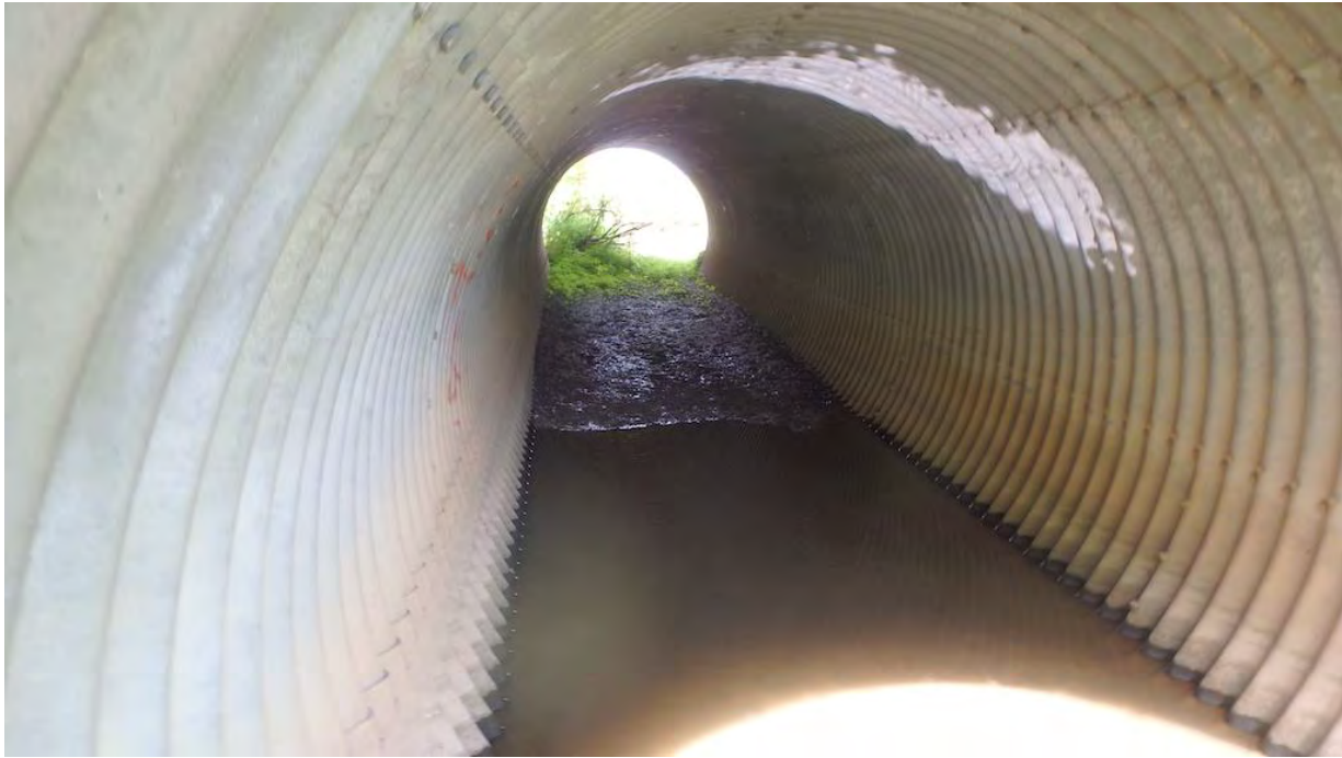
Figure 7 North Barrel, Looking East
