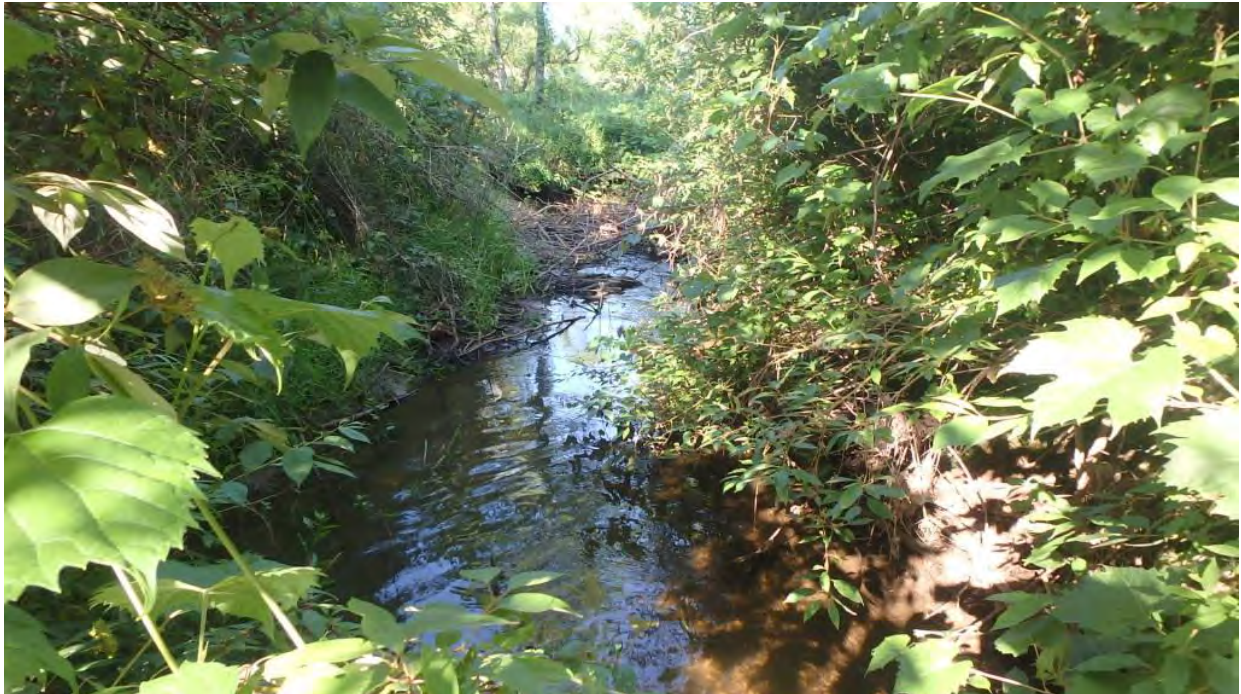
Figure 6 Downstream, Note Blockage at Downstream End
