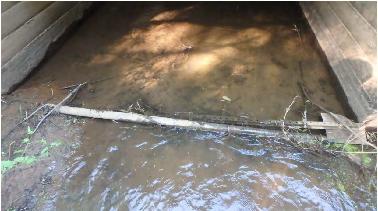
Figure 8 Gas Line at Inlet
