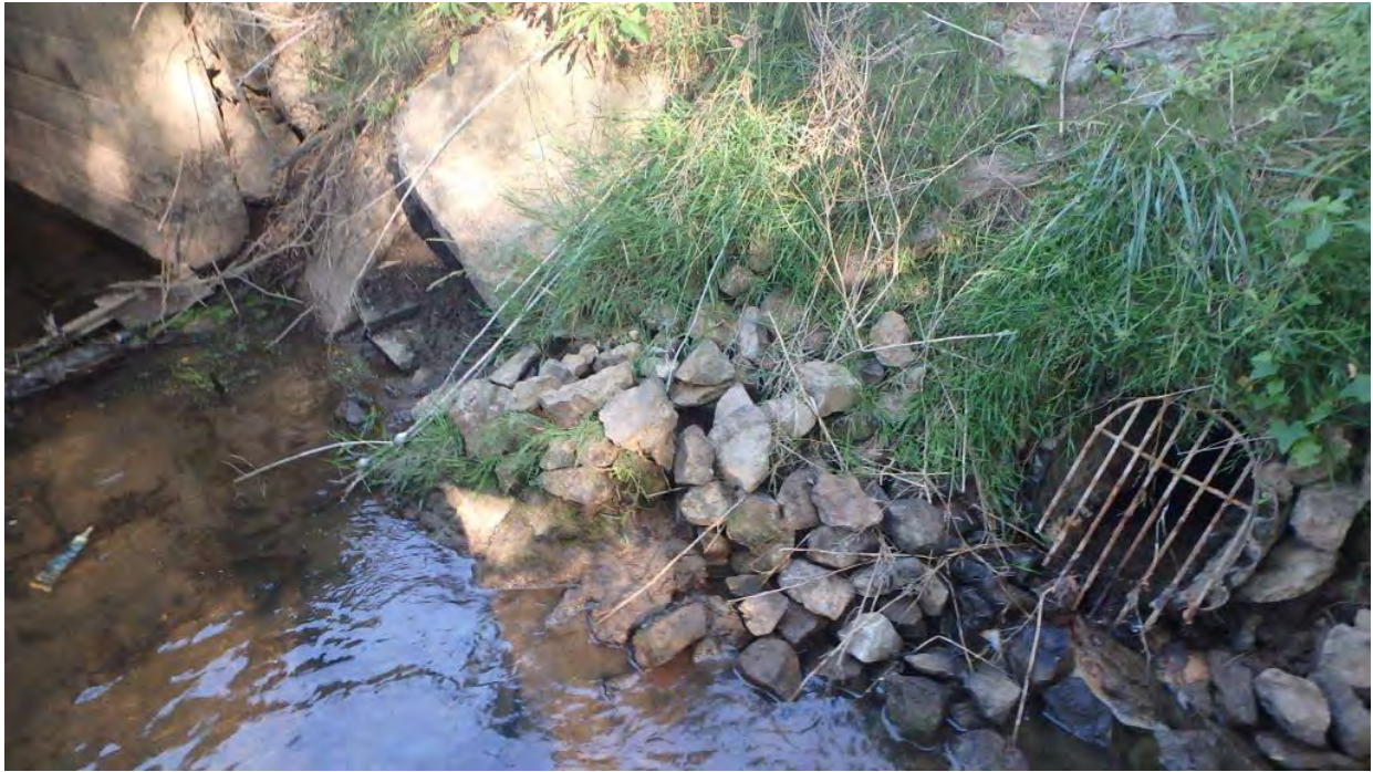
Figure 9 Drain Outlet at Northeast Quadrant
