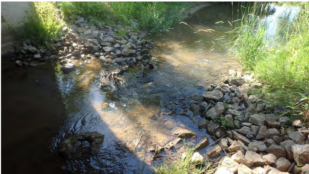
Figure 6 Riprap Build Up at Outlet
