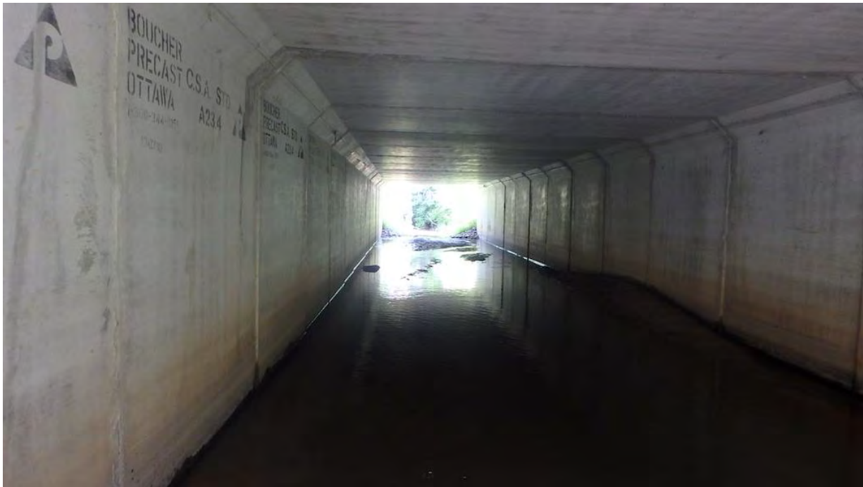
Figure 6 Barrel, Looking South
