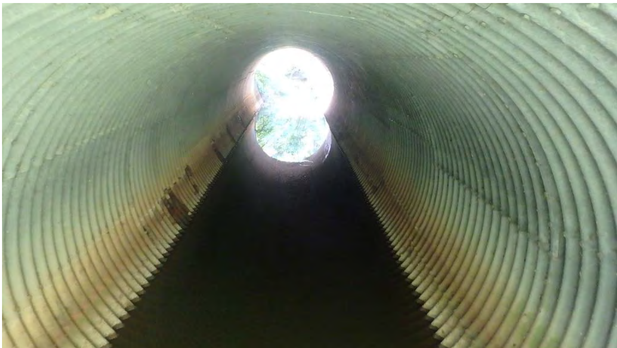
Figure 6 Barrel, Looking South
