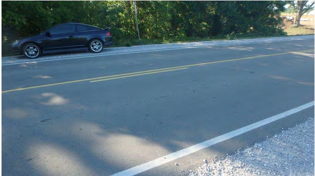
Figure 12 Asphalt Wearing Surface
