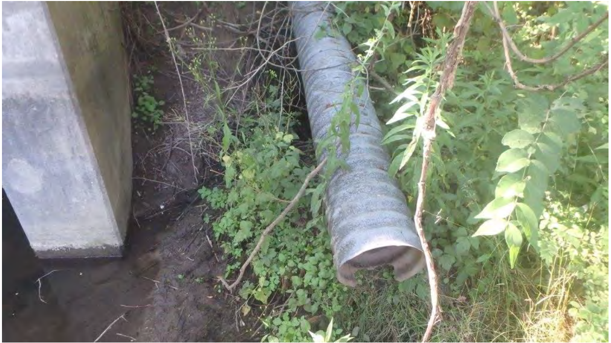
Figure 13 Drain at Outlet
