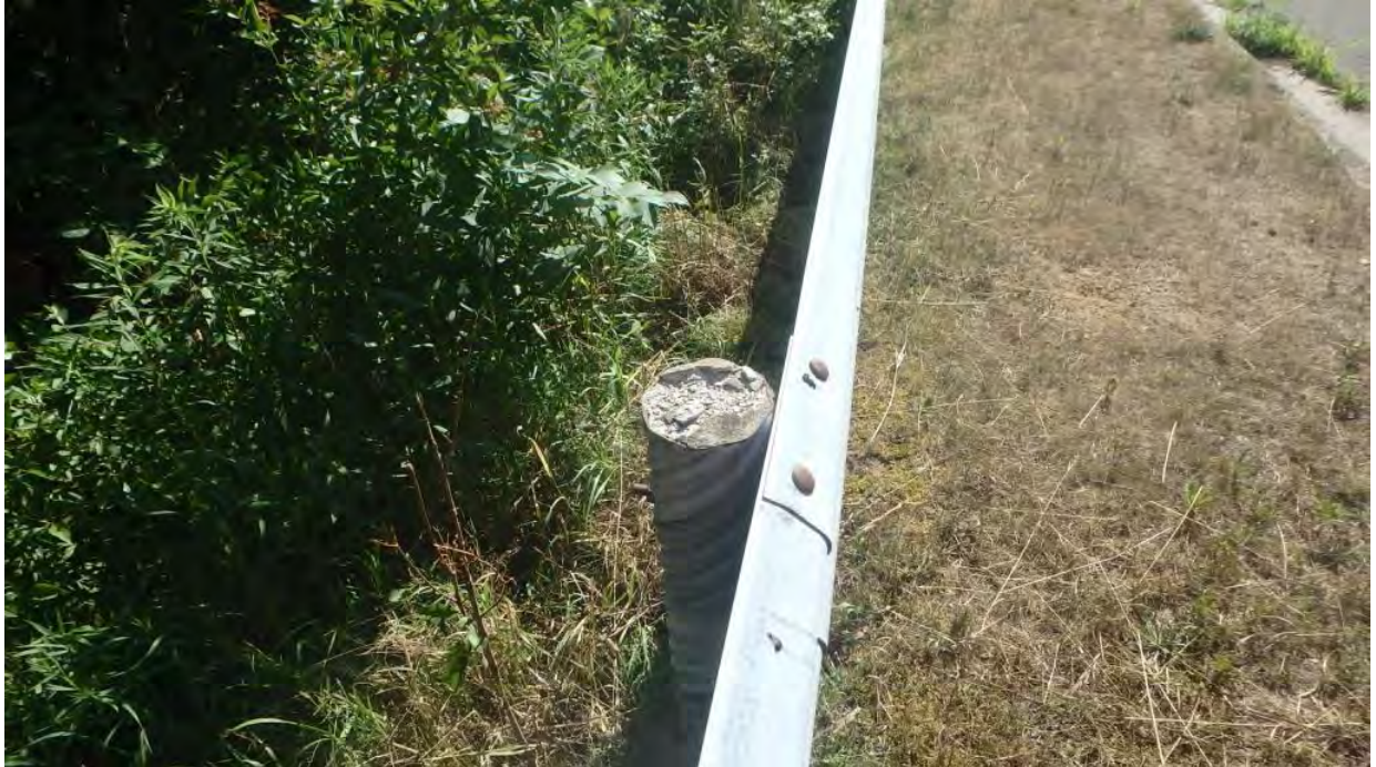
Figure 14 Typical Barrier Post Filled with Concrete
