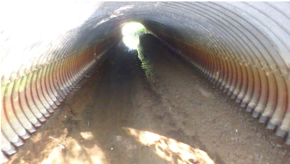
Figure 8 Barrel, Looking West
