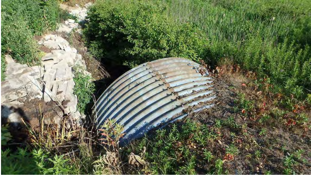
Figure 9 West Culvert Top
