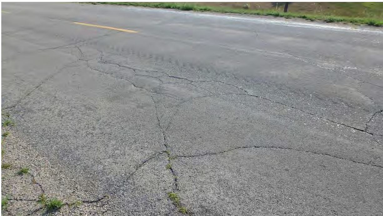
Figure 8 Cracking on Wearing Surface
