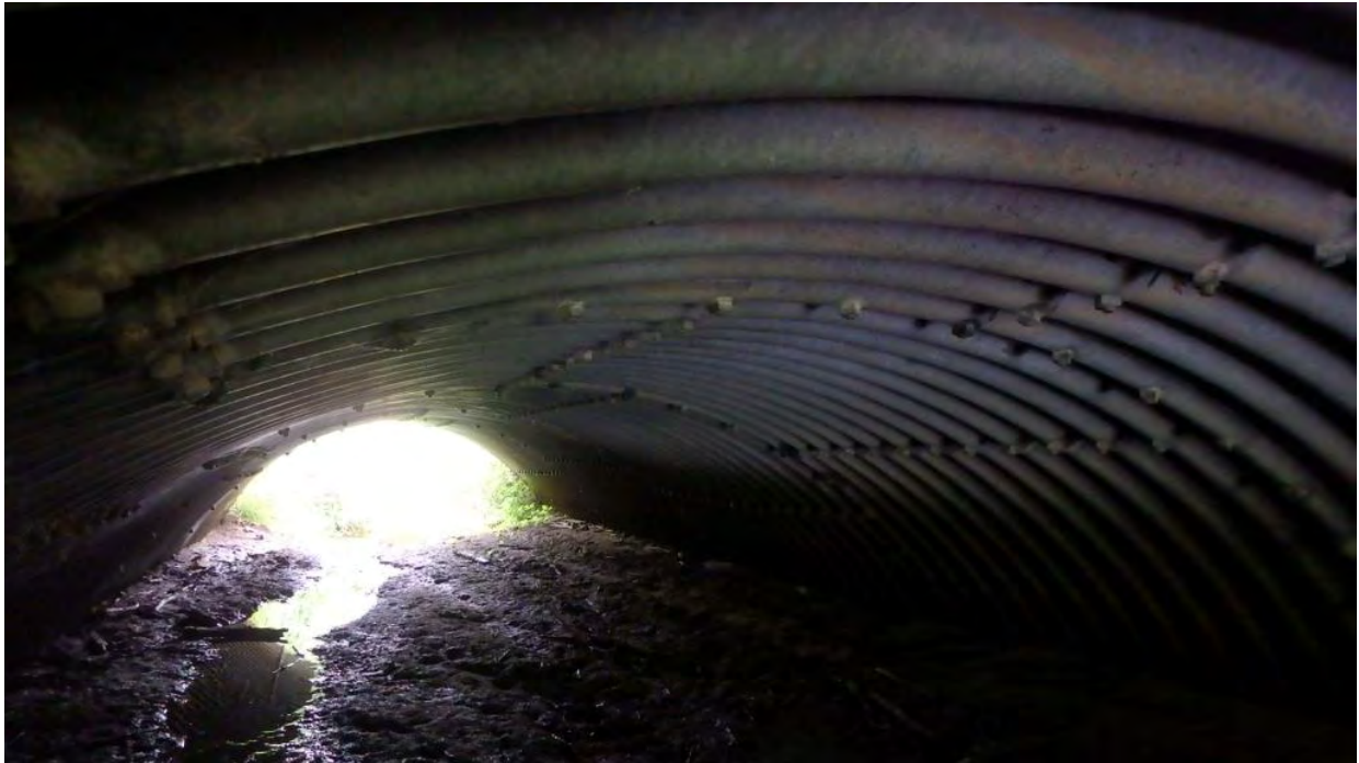
Figure 8 Deflection of Barrel
