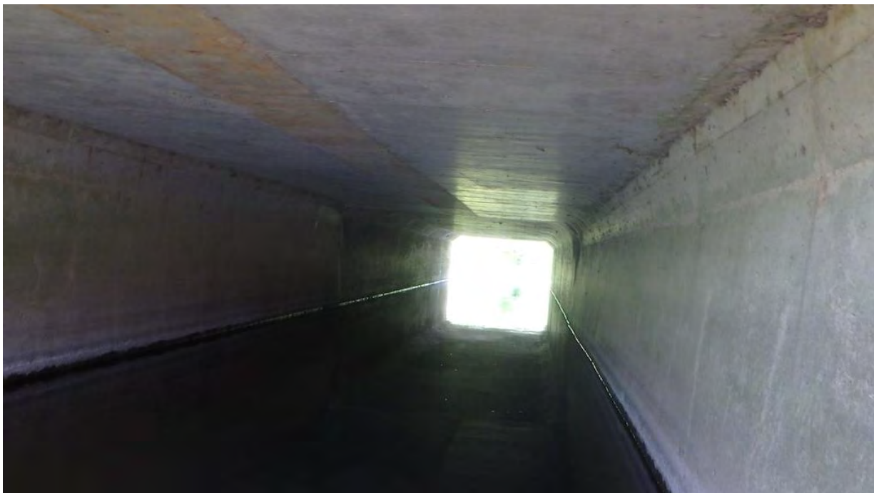
Figure 8 Barrel, Looking South
