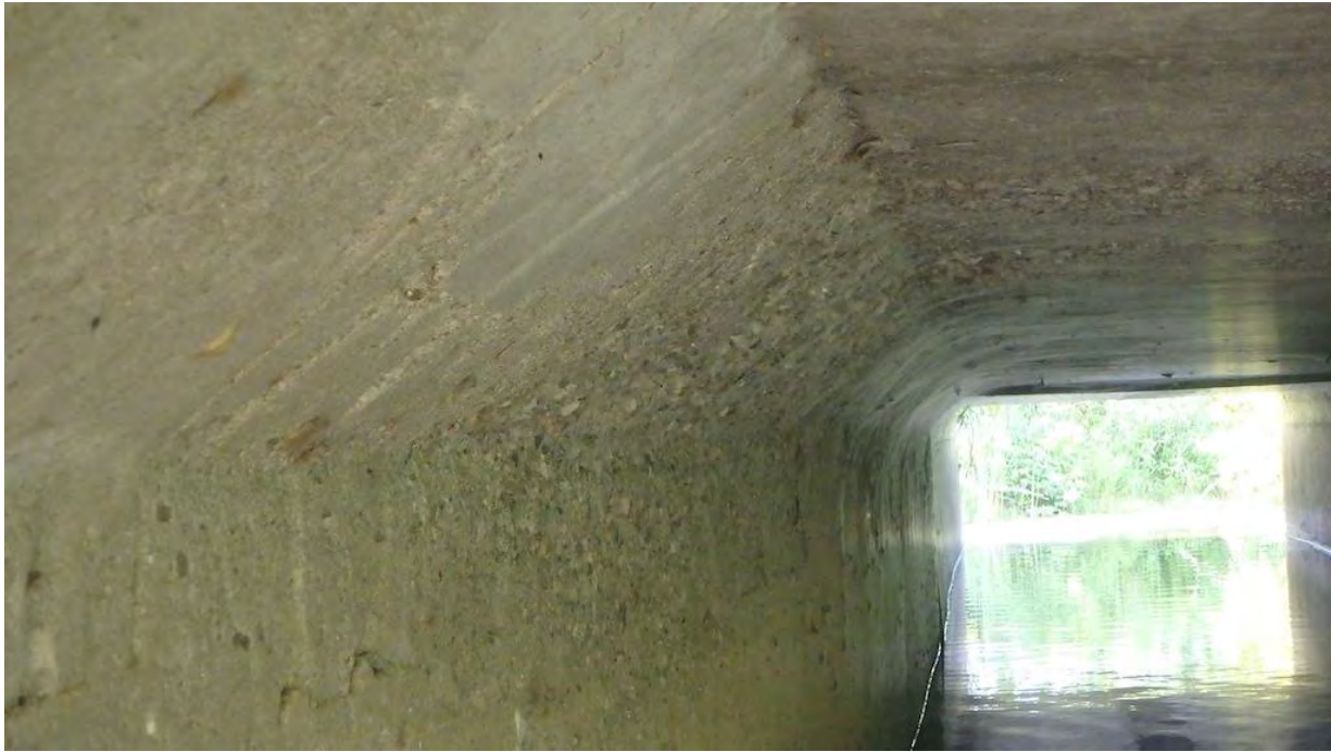
Figure 9 Typical Scaling in Barrel
