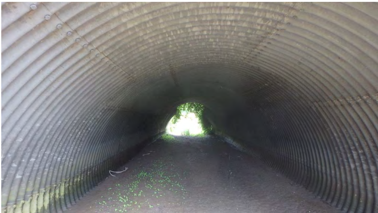
Figure 8 Barrel, Looking West
