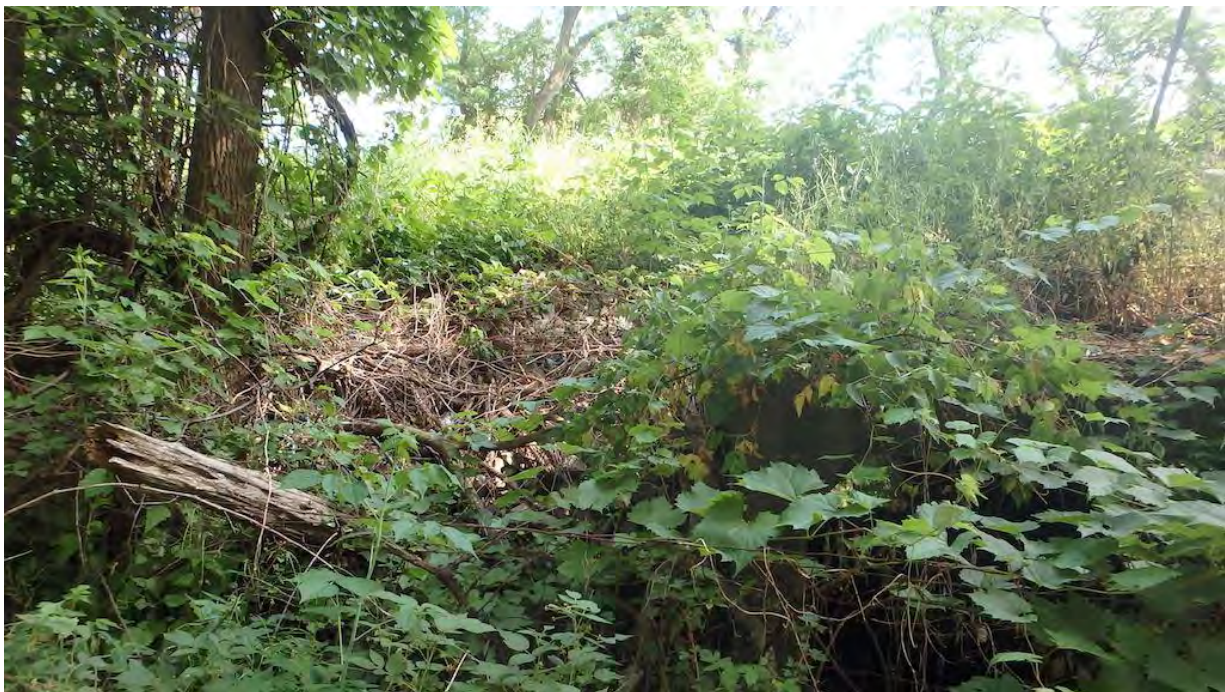
Figure 8 Minor Erosion at Northwest Quadrant
