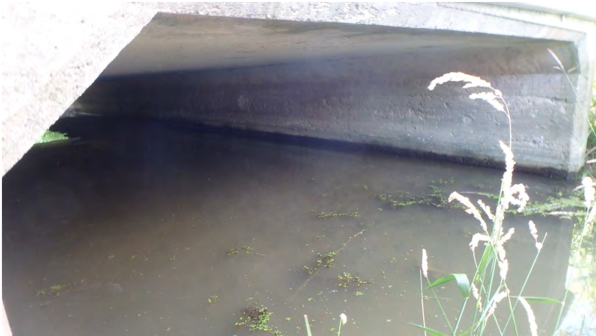
Figure 8 West Culvert Wall
