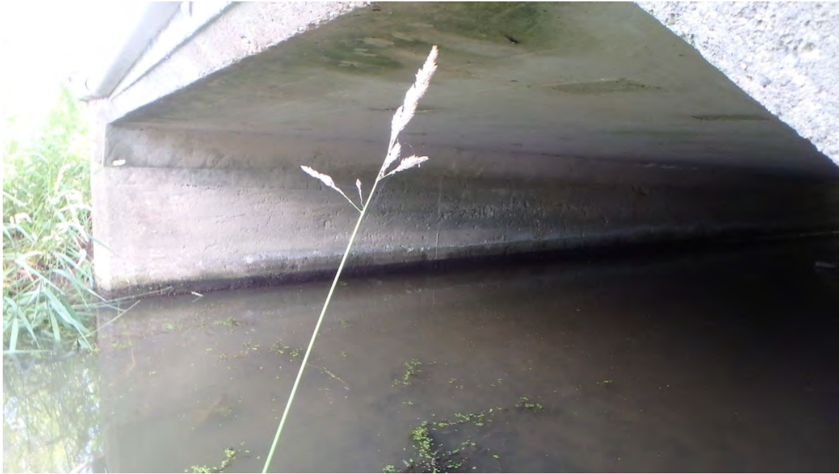
Figure 7 East Culvert Wall
