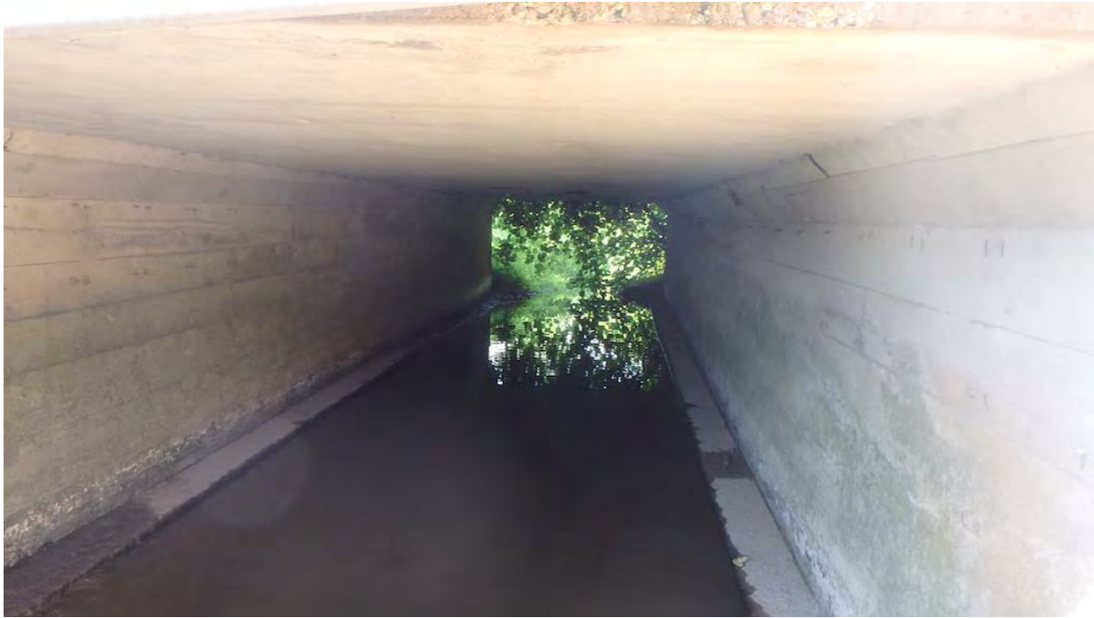
Figure 7 Barrel, Looking South
