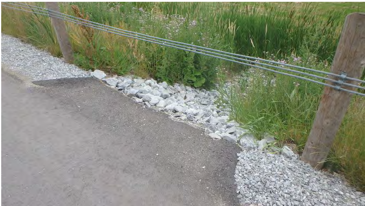
Figure 8 Typical Asphalt Spillway
