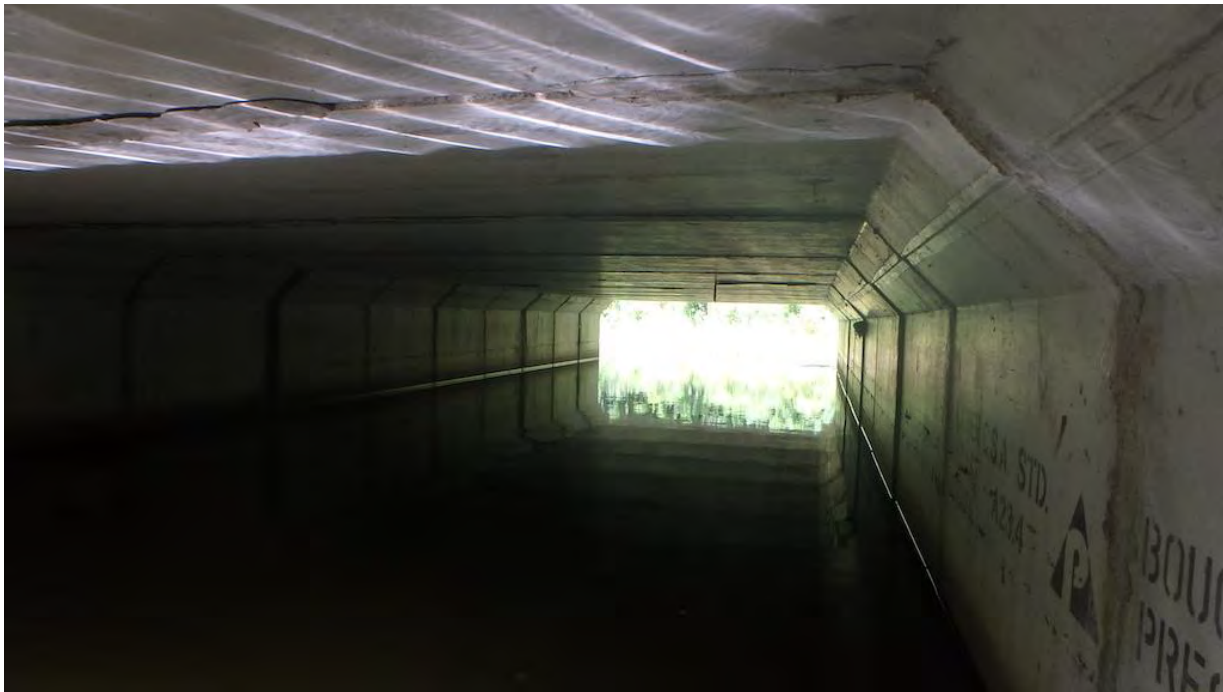
Figure 8 Barrel, Looking West
