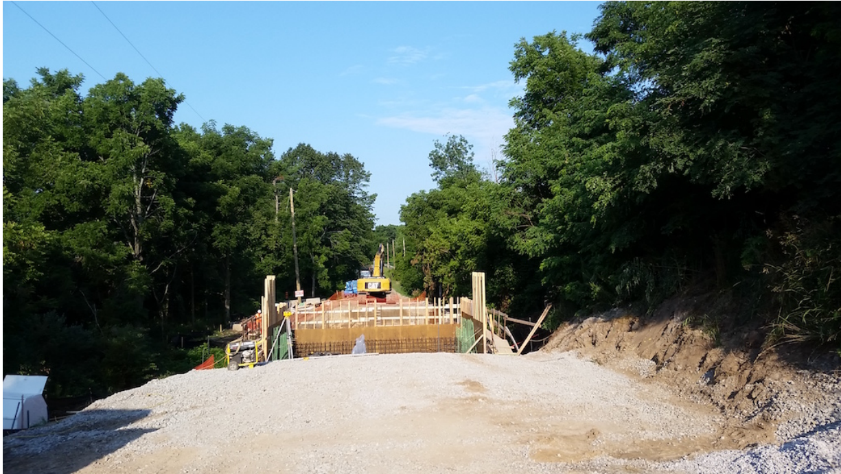
Figure 1 Bridge Under Construction, 2016
