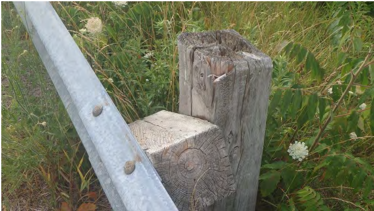
Figure 15 Typical Approach Barrier Post
