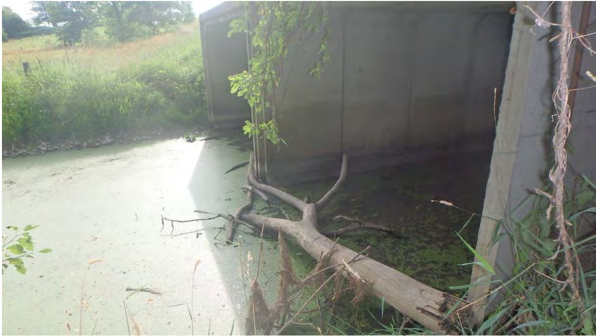
Figure 12 Fallen Tree at West Inlet Barrel
