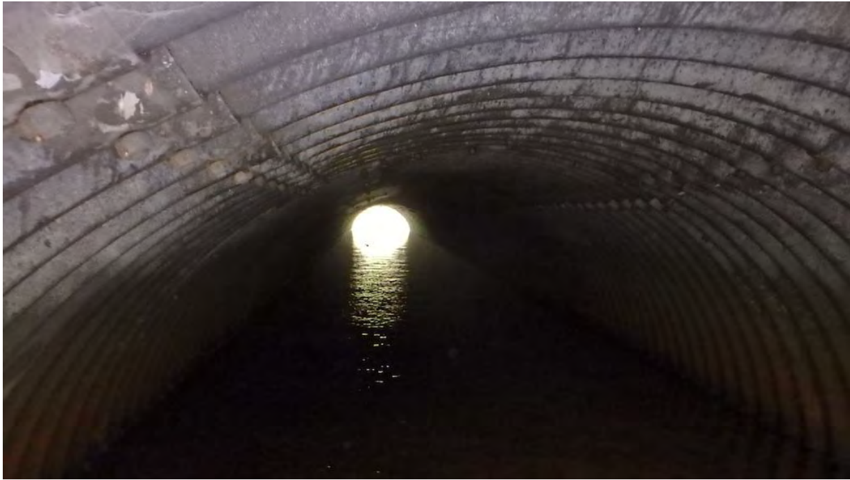
Figure 7 Barrel, Looking South
