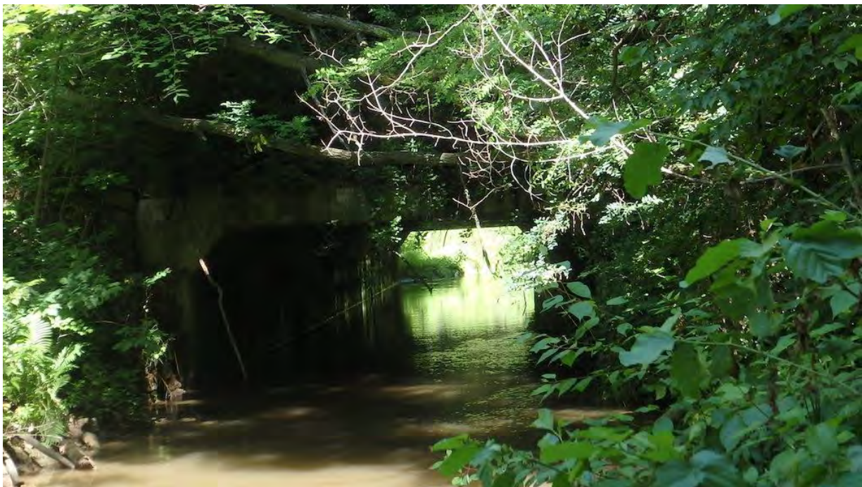
Figure 6 South Culvert Fascia
