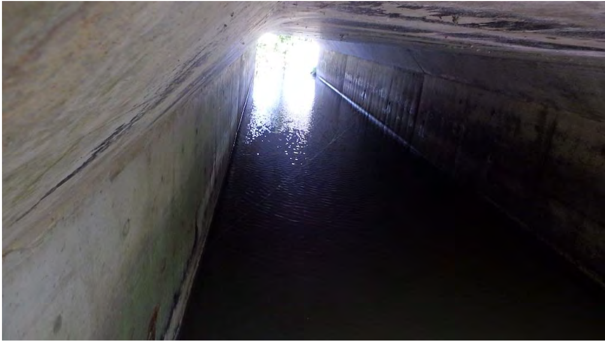
Figure 7 East Barrel, Looking North
