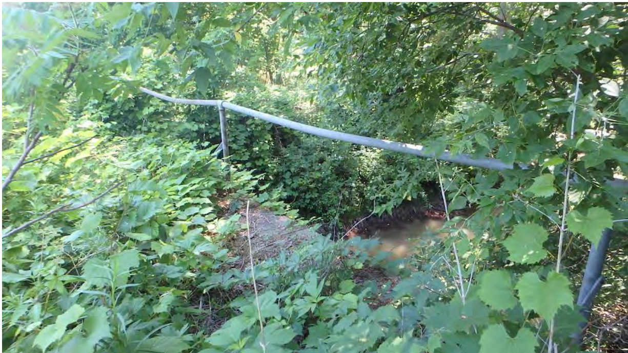
Figure 12 Handrail on South Culvert Top
