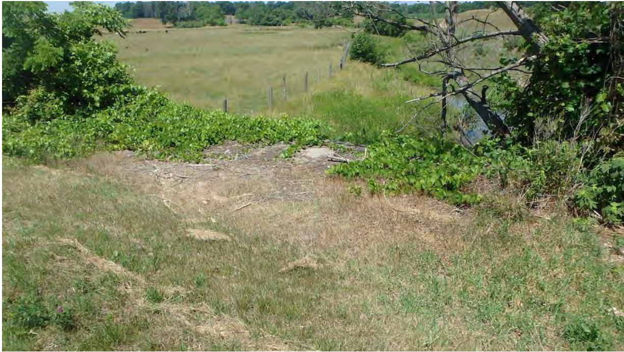
Figure 11 North Culvert Top
