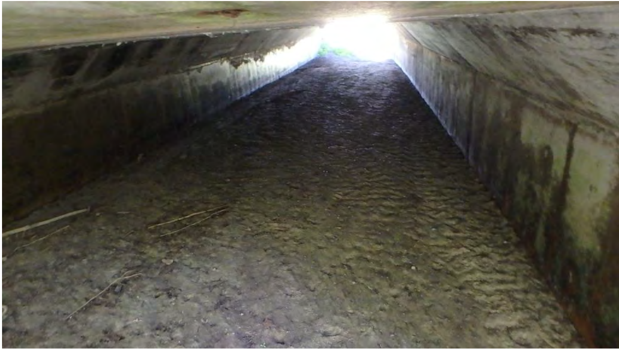
Figure 9 West Barrel, Looking North
