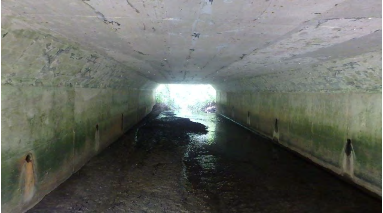
Figure 6 Barrel, Looking East
