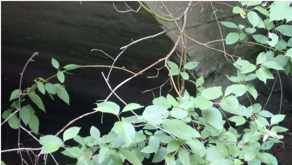
Figure 8 Deterioration of Corners
