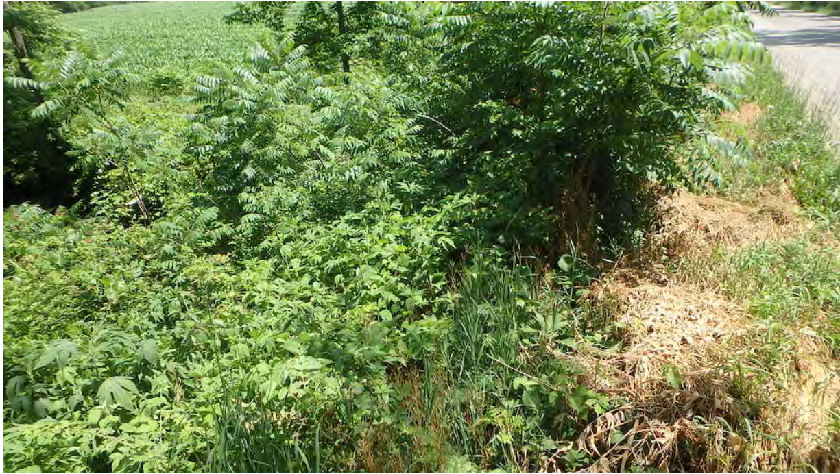
Figure 3 Inlet – Culvert Top
