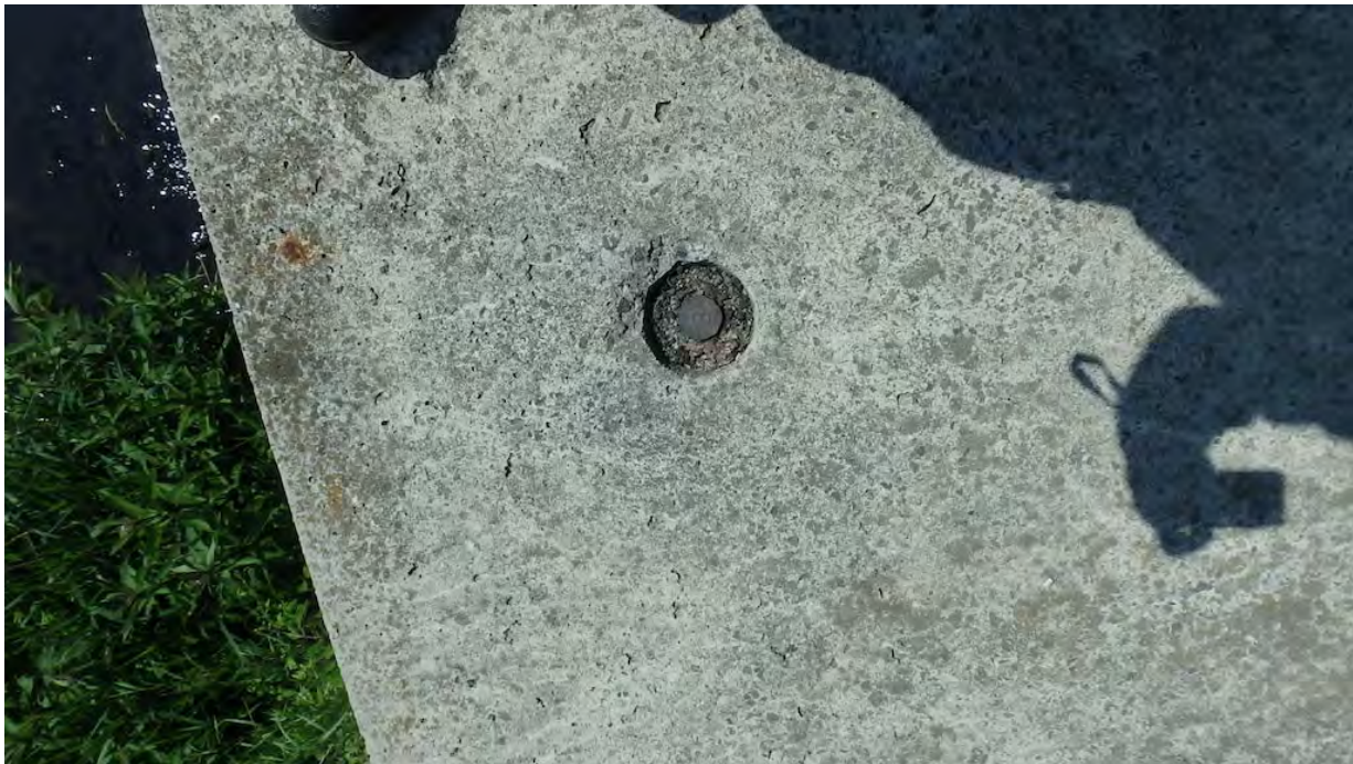
Figure 10 Lifting Lug on Culvert Top
