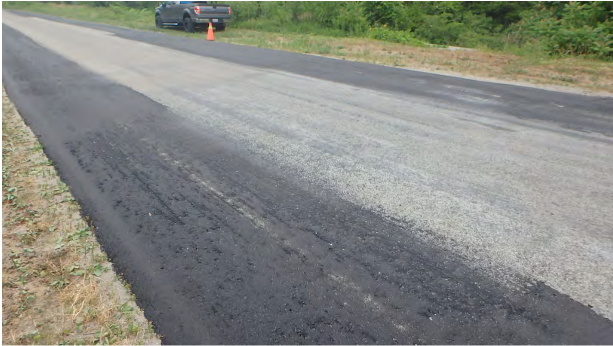
Figure 11 Wearing Surface, Patched
