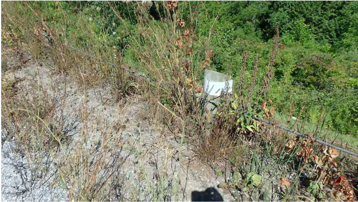
Figure 5 Single Cable Guiderail at North
