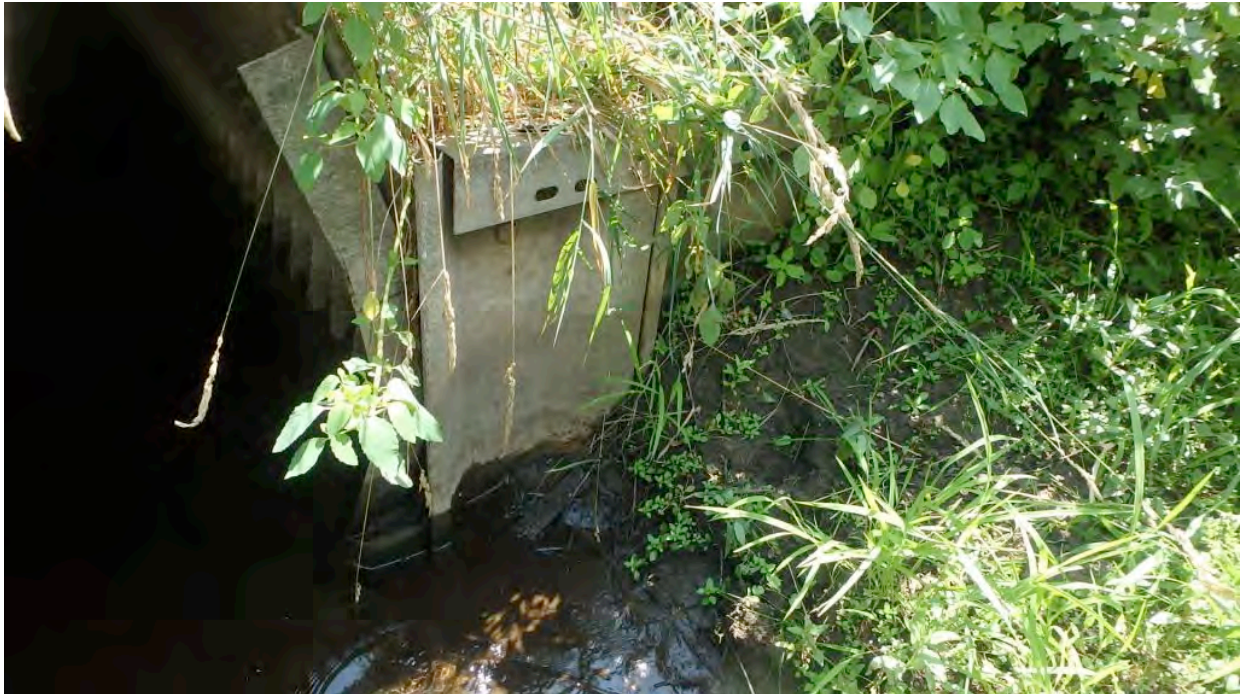
Figure 10 Retaining Walls at All Quadrants
