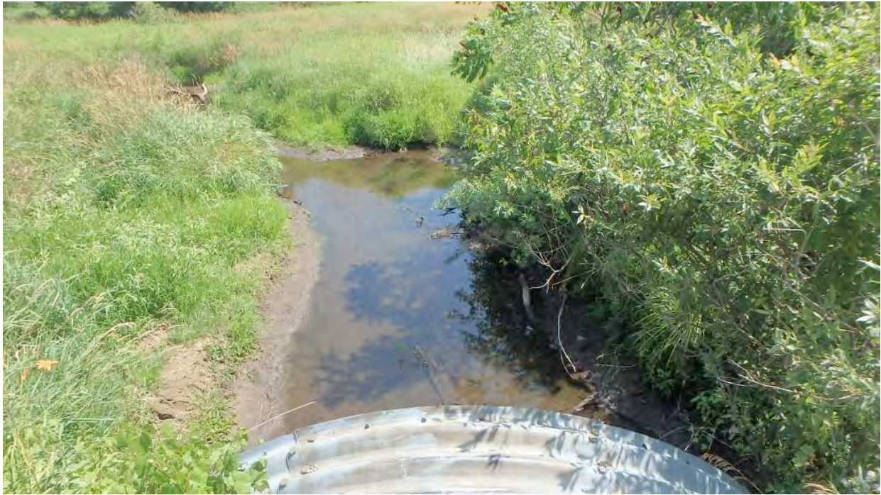
Figure 5 Upstream (Looking East)
