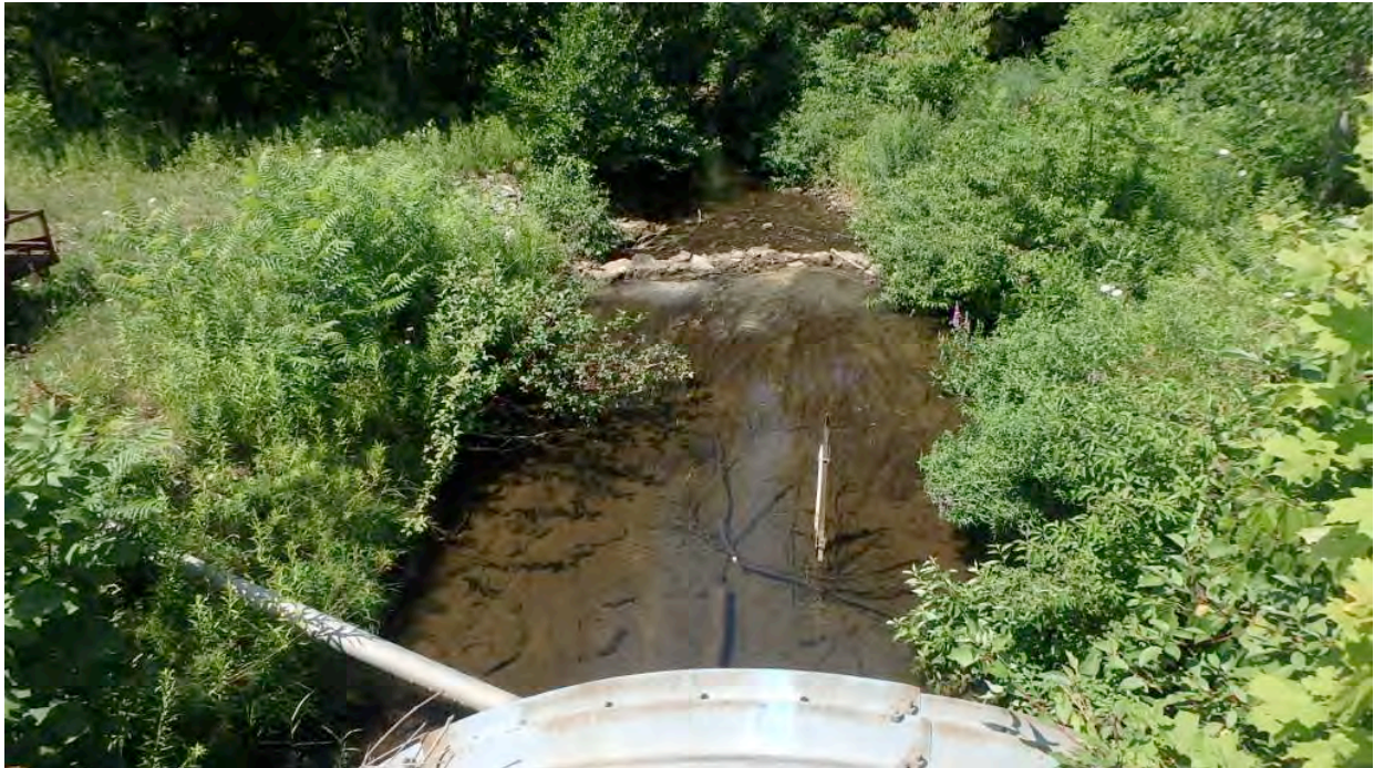
Figure 6 Downstream (Looking West)
