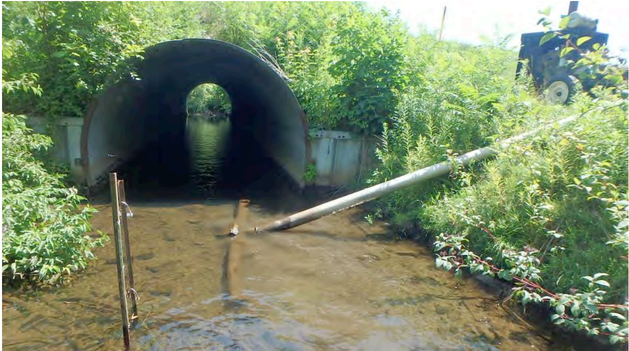
Figure 10 Irrigation Pipe in Waterway
