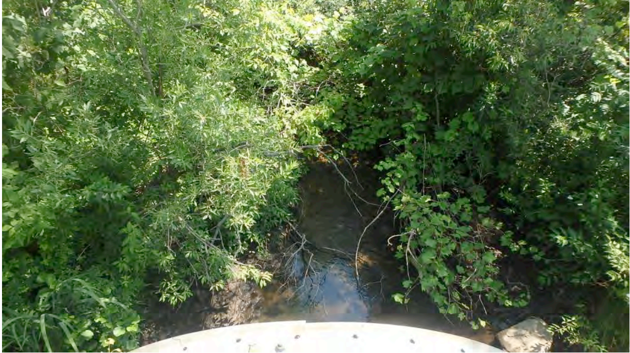
Figure 5 Upstream (Looking East)
