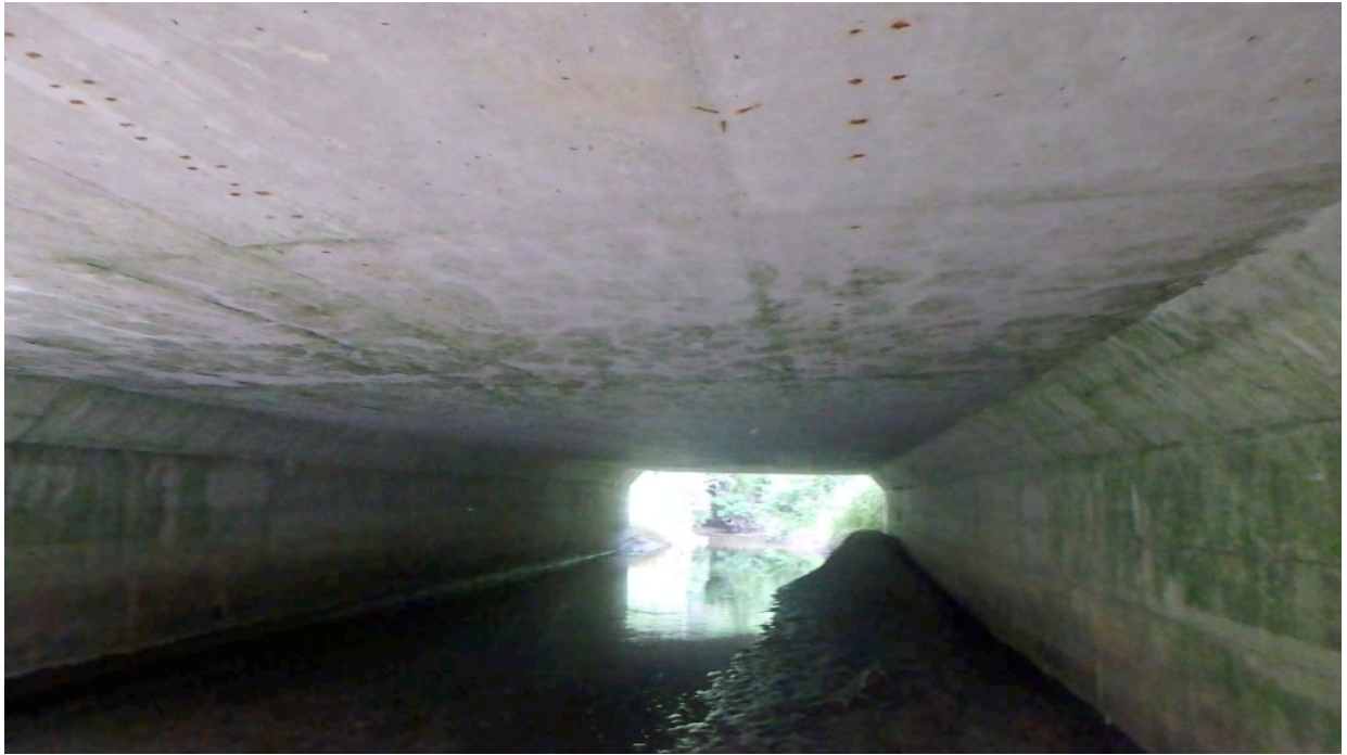
Figure 7 Barrel, Looking North
