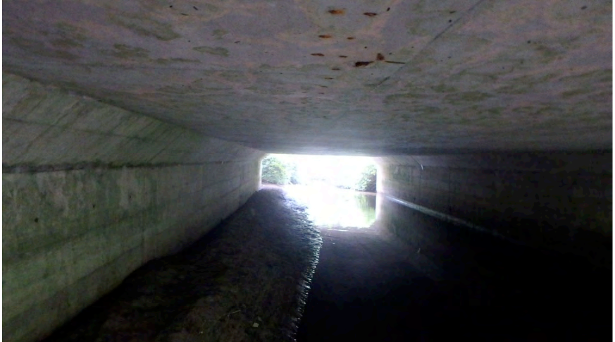
Figure 8 Barrel, Looking South
