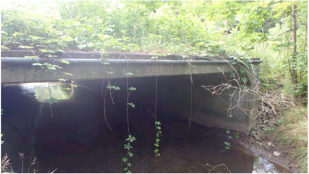
Figure 11 Utility Line on Fascia
