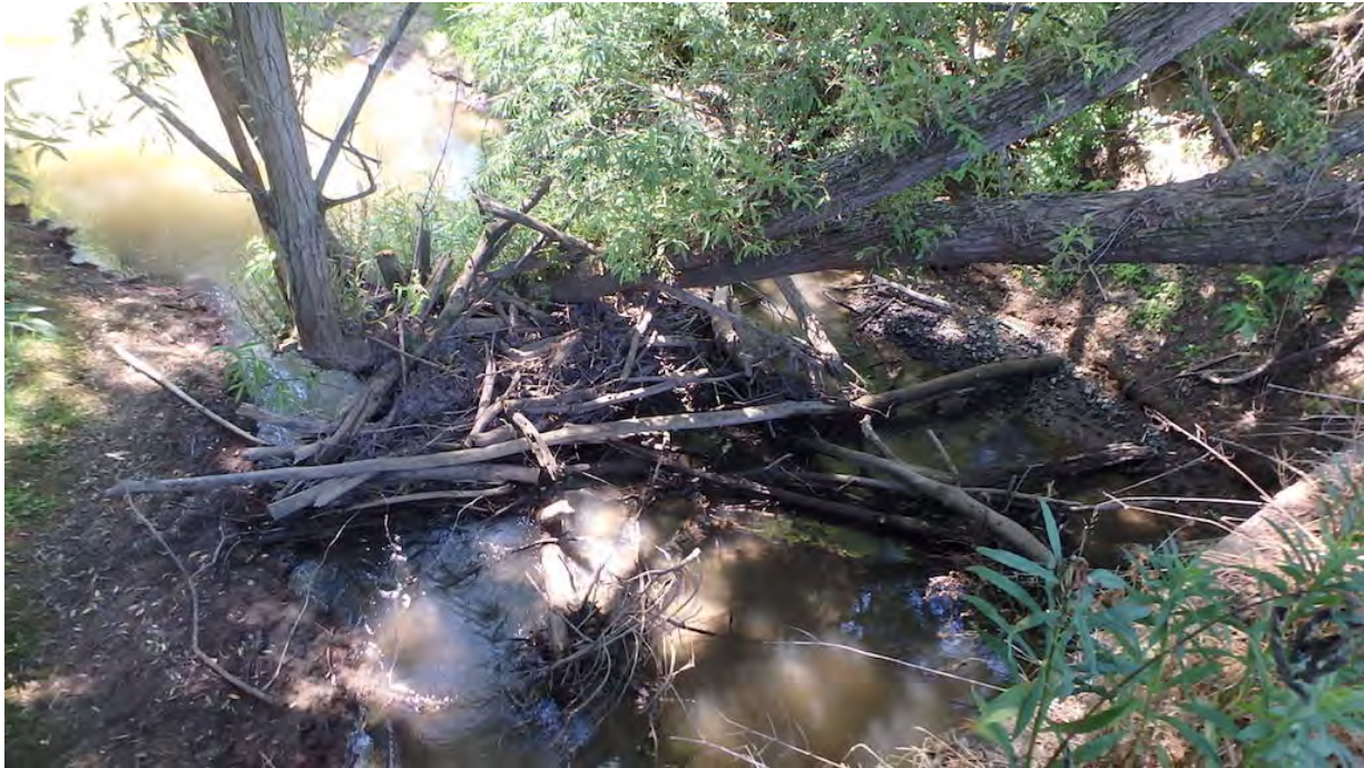
Figure 3 Debris Blocking Outlet
