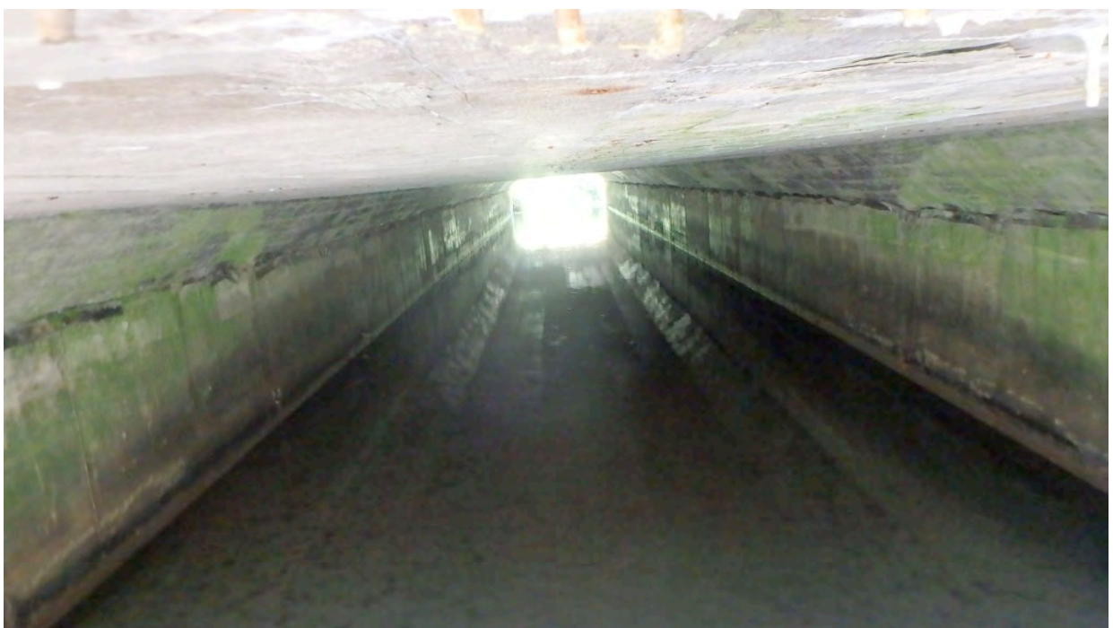
Figure 6 Barrel, Looking South
