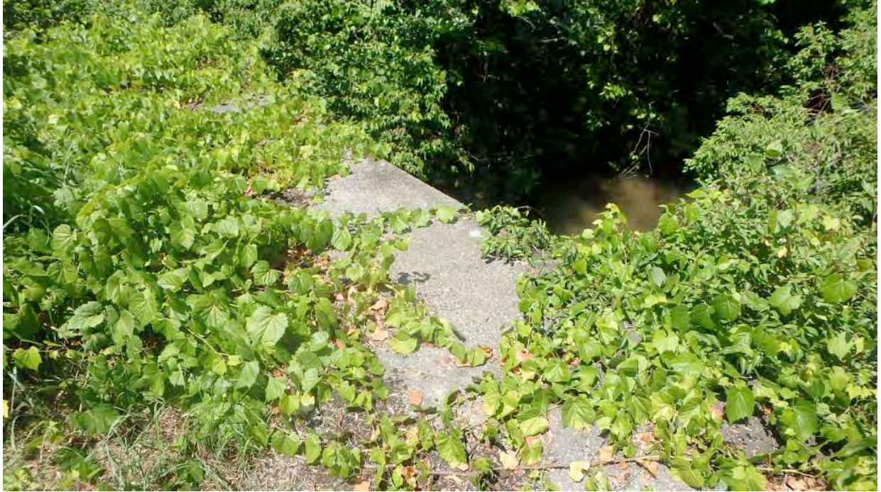
Figure 3 North Culvert Top
