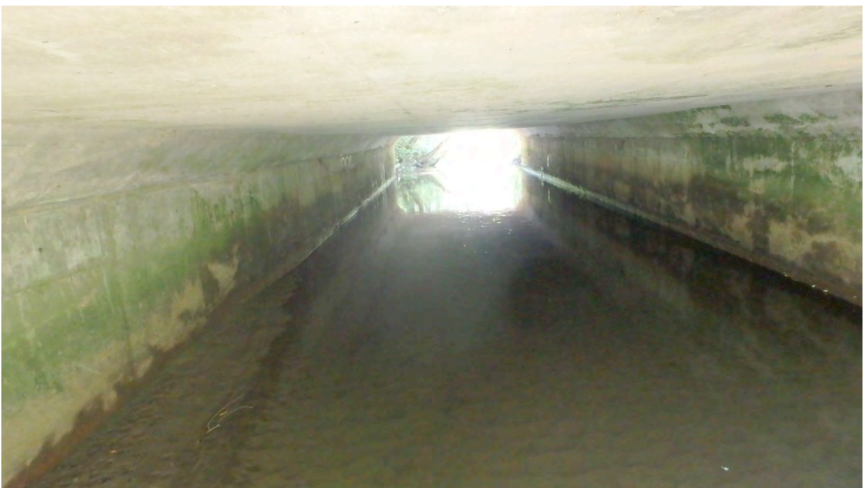
Figure 8 Barrel, Looking South
