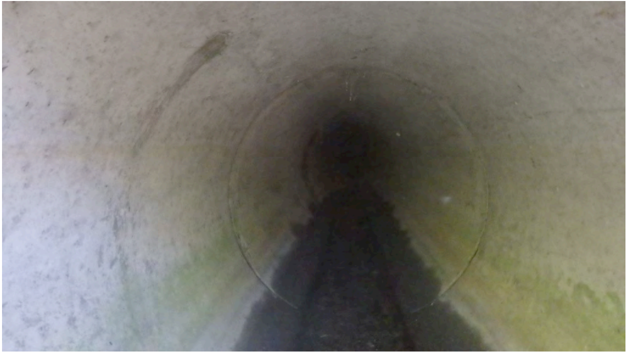
Figure 7 South Pipe Barrel
