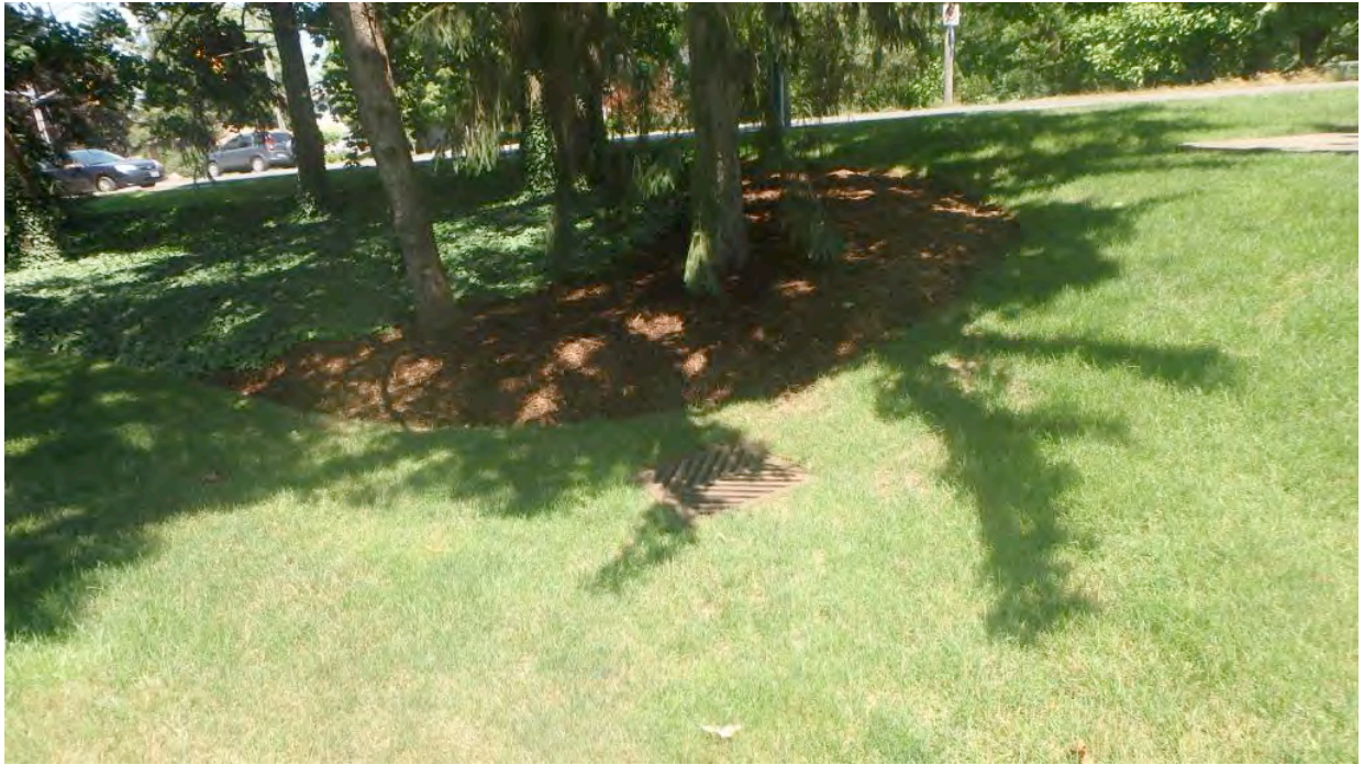
Figure 9 Catch Basin at Outlet
