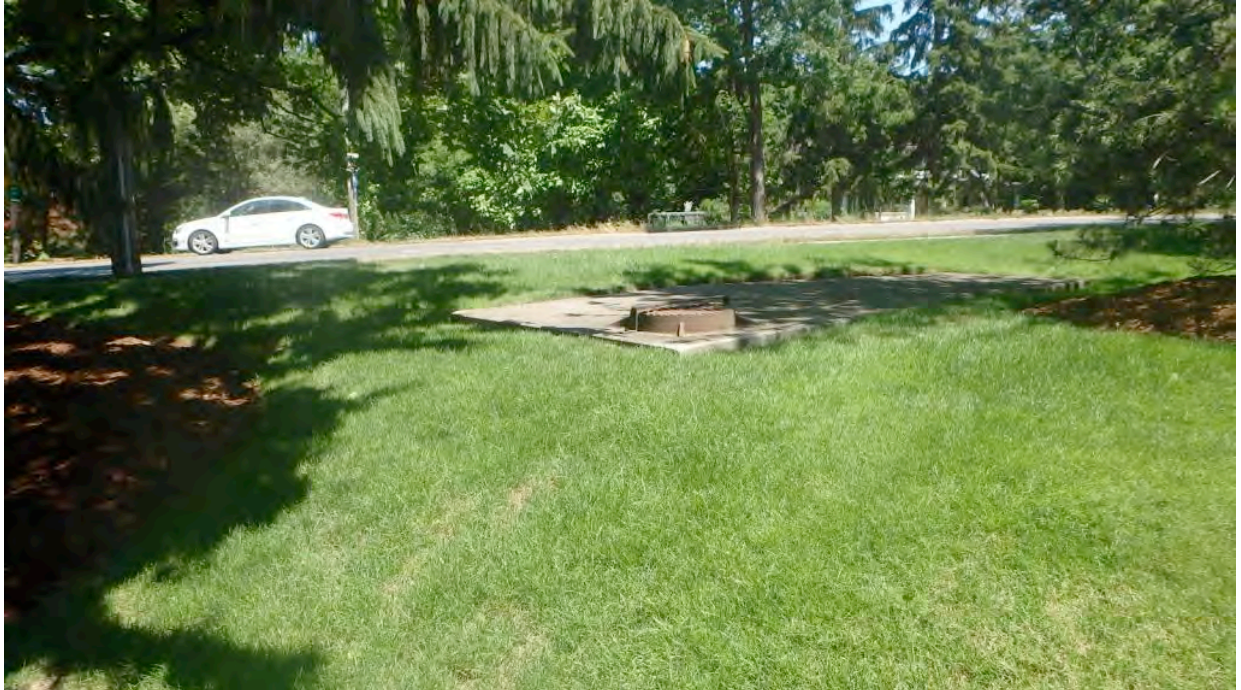
Figure 10 Manhole at Outlet
